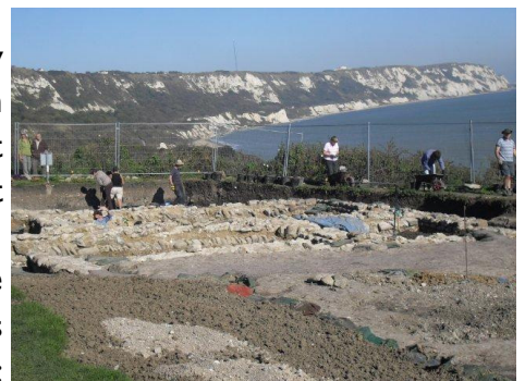
Work in Progress at East Wear Bay
